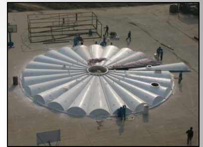
60' dia. hot clarifier covers for FLS/SNC Lavalin
