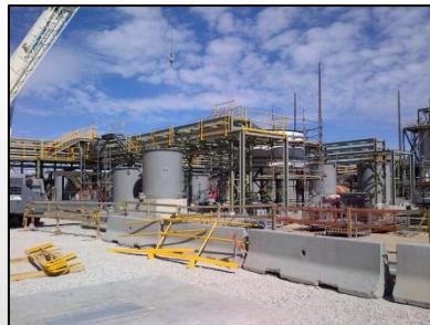
FRP tanks for FMI Arizona
