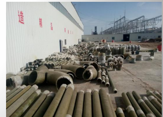
On site installation
