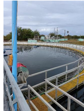
Two 120' diameter trough, weir and drop out systems for Puerto Rico
