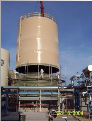
350,000 gal. potable water tank Arizona
