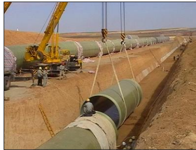
19 km. of 3.1 M water pipe
