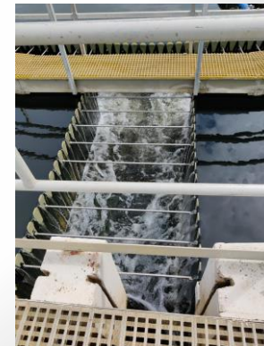
Two 120' diameter trough, weir and drop out systems for Puerto Rico
