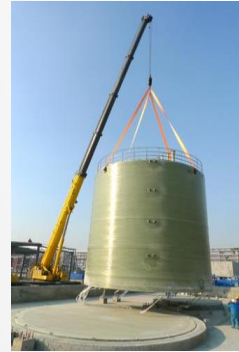
Demold the tank body and move it to the concrete foundation
