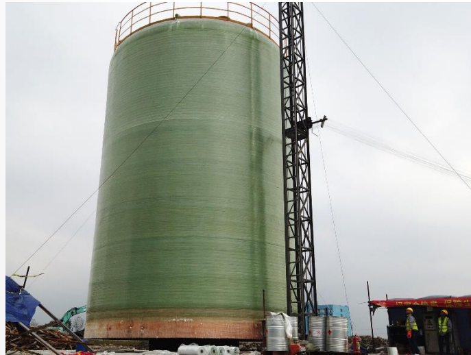
Wind the structural layer
