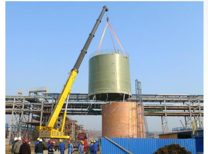
Demolding after curing
