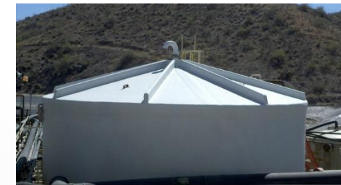
Come into service after hydrostatic test
