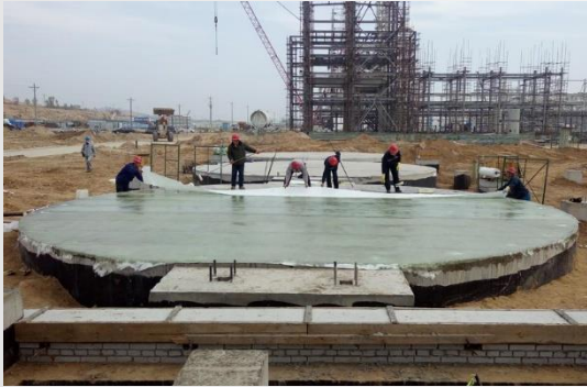
Make tank bottom on the concrete foundation
