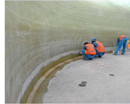
Bond the tank body and heads
