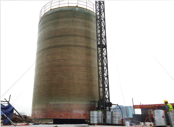
Make Corrosion Barrier
